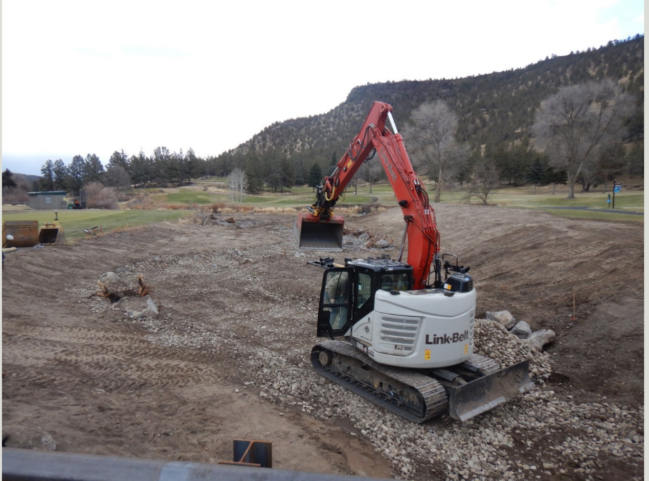
Grading river rock materials for the final channel elevation; October 2022
