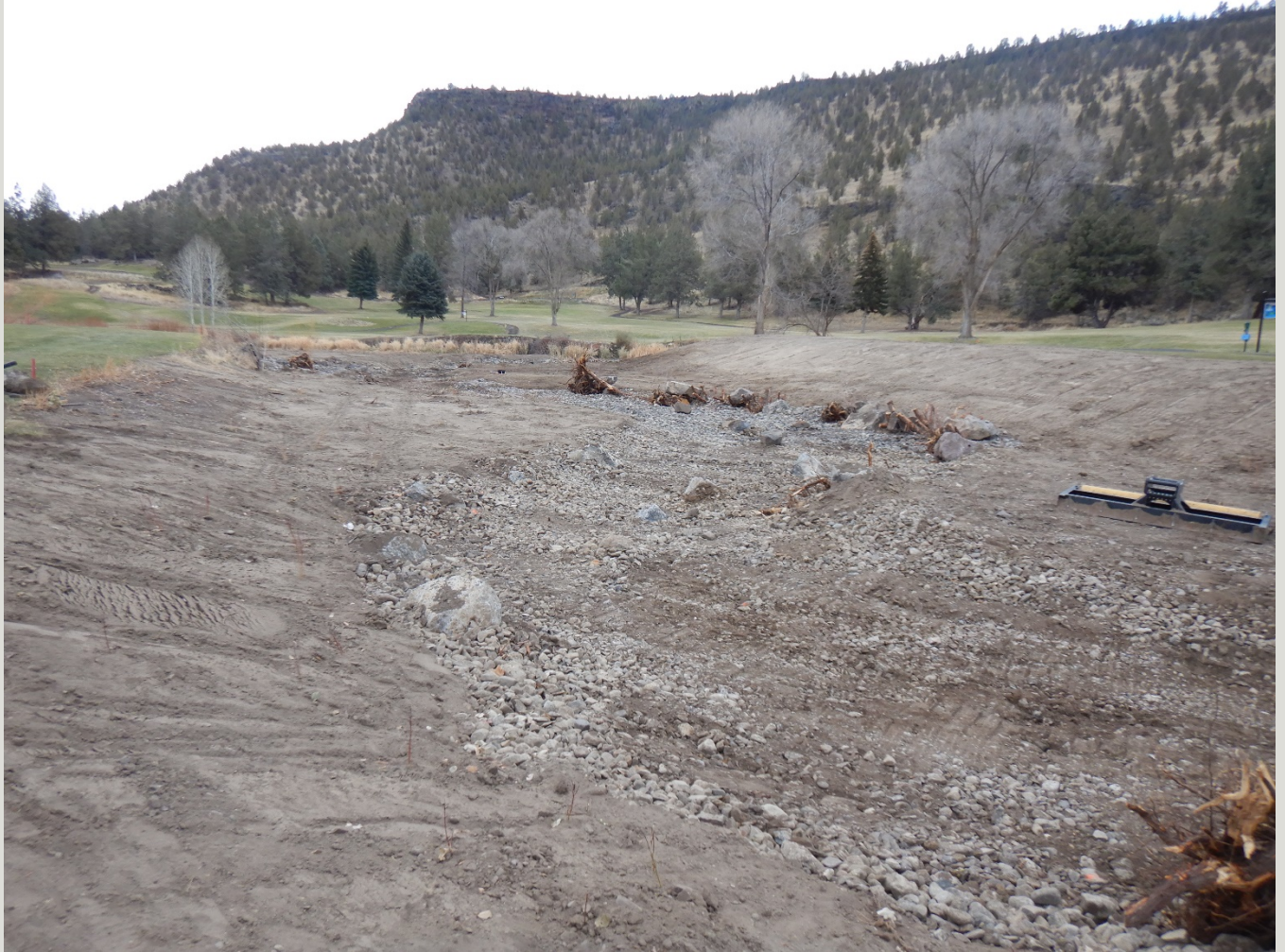
Final slope grades and channel alignment on Ochoco Creek
