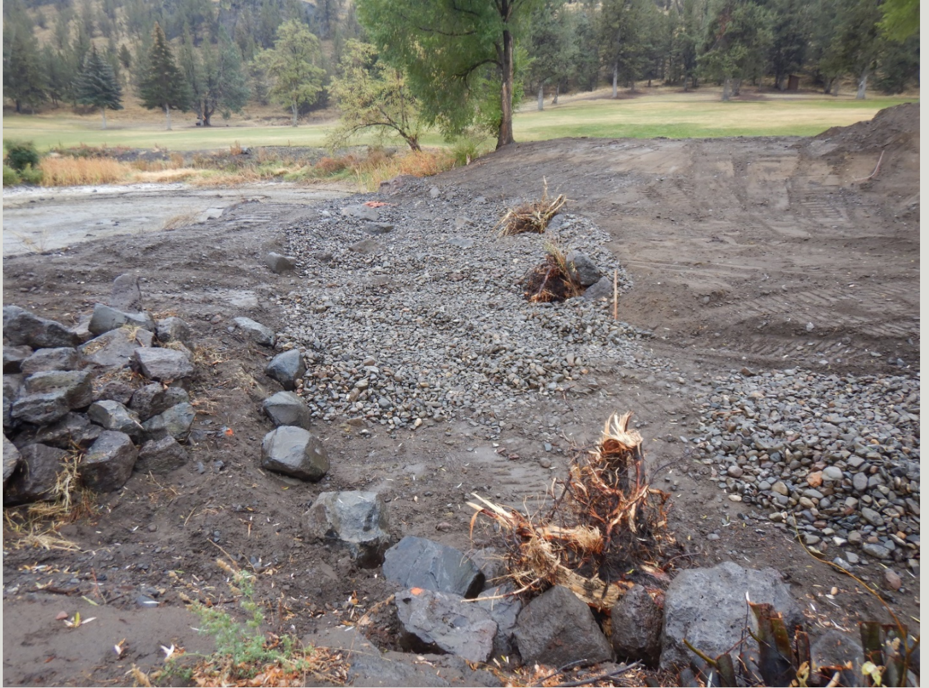
Final channel configuration, bed materials, and juniper log structures for the new roughened riffle fish passage project on Ochocho Creek.
